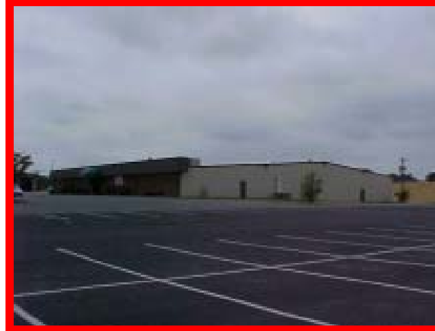
23,000 S.F. 631 Cinema Dr., Kernersville, NC PIEDMONT LANES BOWLING ALLEY
