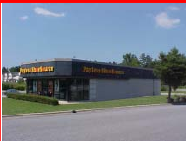
3000 S.F. 2726 N. Main St., High Point, NC RETAIL OUTLET
