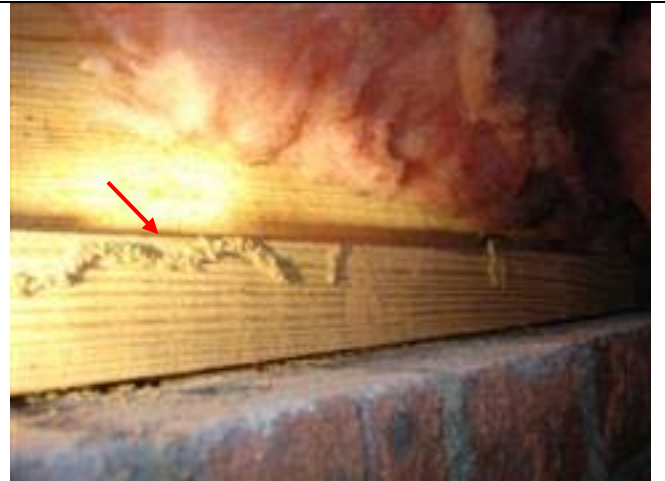
Insect tunneling on left front floor sills.
