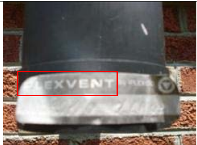
PLEXVENT exhaust venting is specifically recalled by the CPSC.
