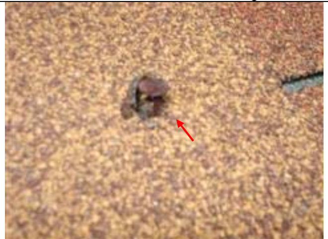
A single nail has “popped” up through shingles over the sun room.
