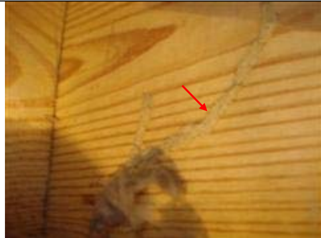
Insect tunneling on left front floor sills.
