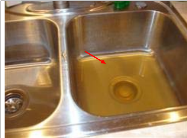
Brownish water from water heater.
